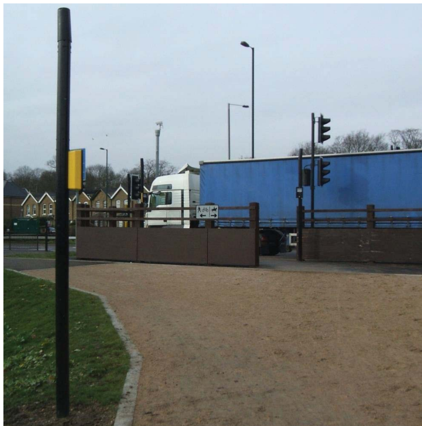
Equestrian facility as installed across Roehampton Vale
